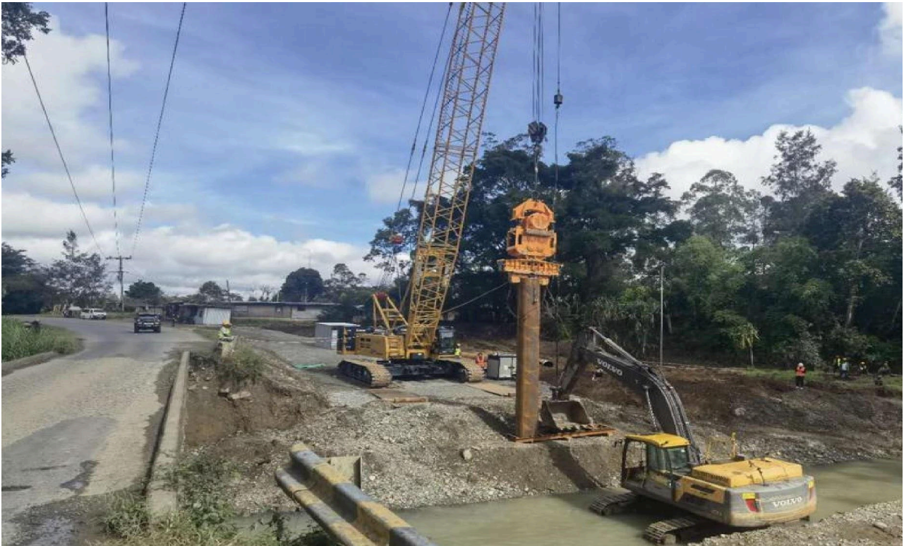
Photo 31: Detour Access Piling Work for Substructure on Bilu Bridge, Jiwaka Section
