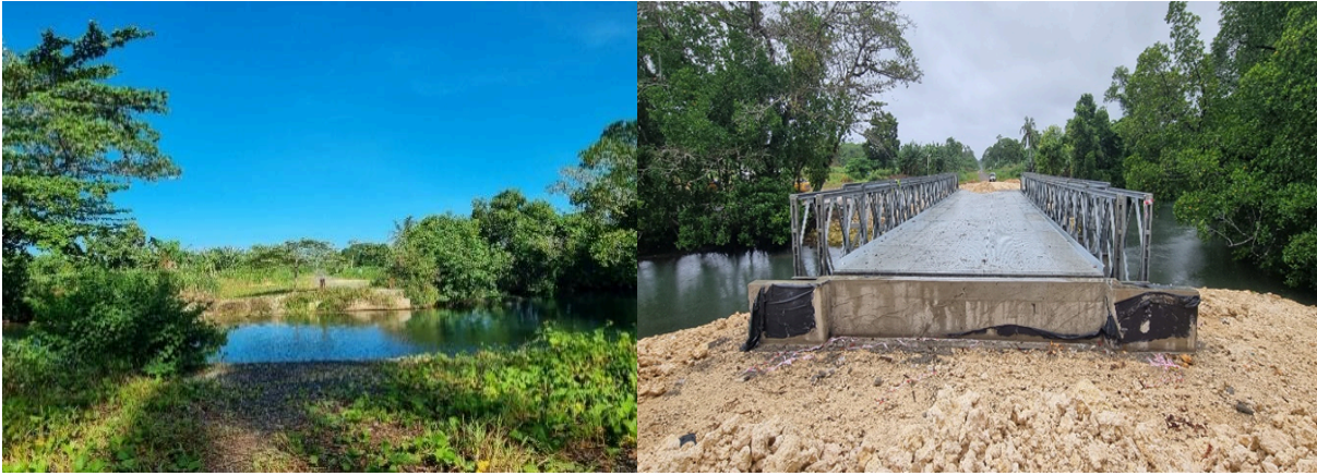
Photo 22: Construction of Soalaba (Karu) Dual Lane Bridge, Boluminsky Highway
