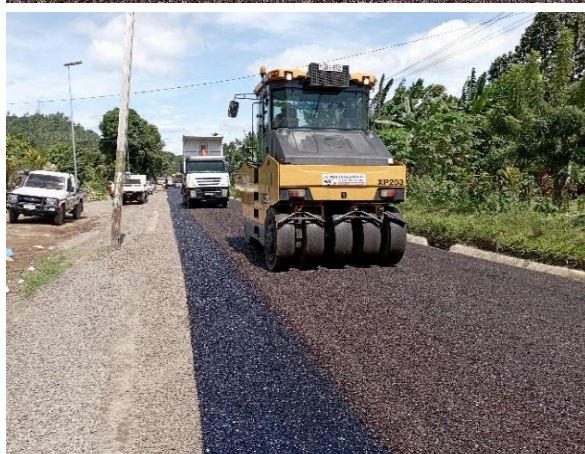
Photo 25: Spreading 14mm chips and 2 nd Coat 14mm at Kimbe Police Barracks
