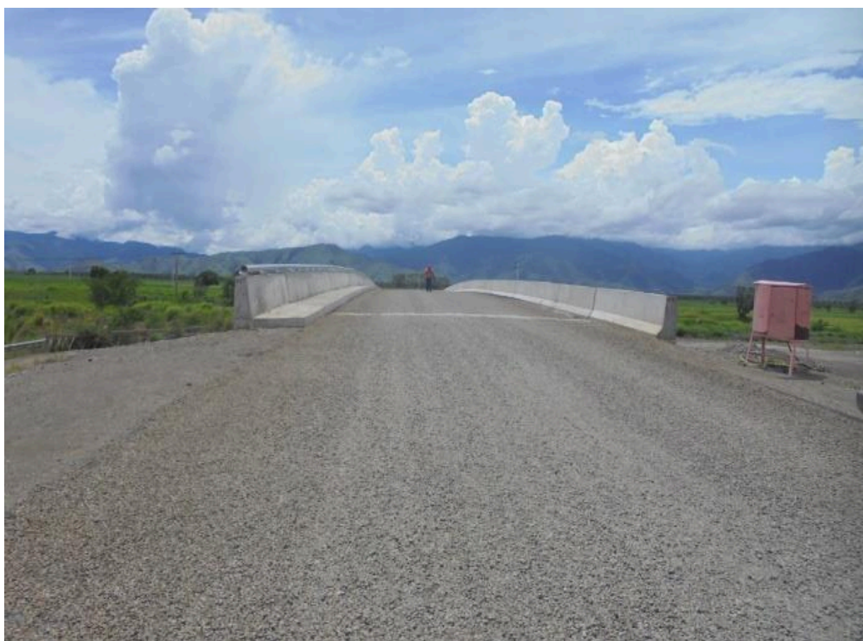
Photo 36: Bora Bridge on the Ramu Highway
