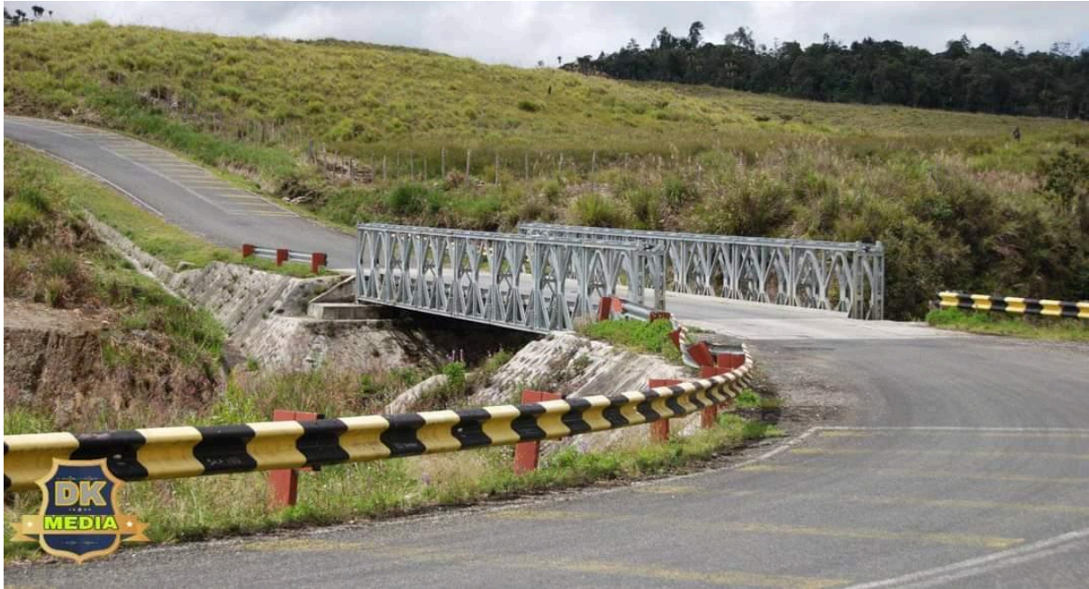
Photo 56: Rural Bailey Bridge Standard delivered on Tambul-Nebilyer District Rural Road under the Multi-Year Rural Bridging Program with United Pacific Bridges Ltd.
