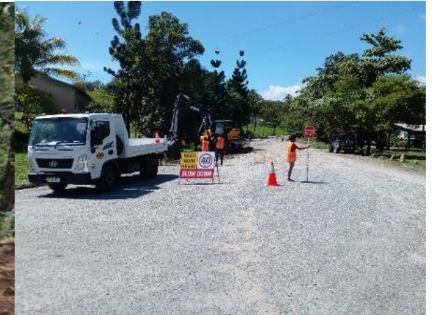
Photo 83: Upgrading and Sealing-Bulolo Junction-Hidden Valley Junction, Bulolo District
