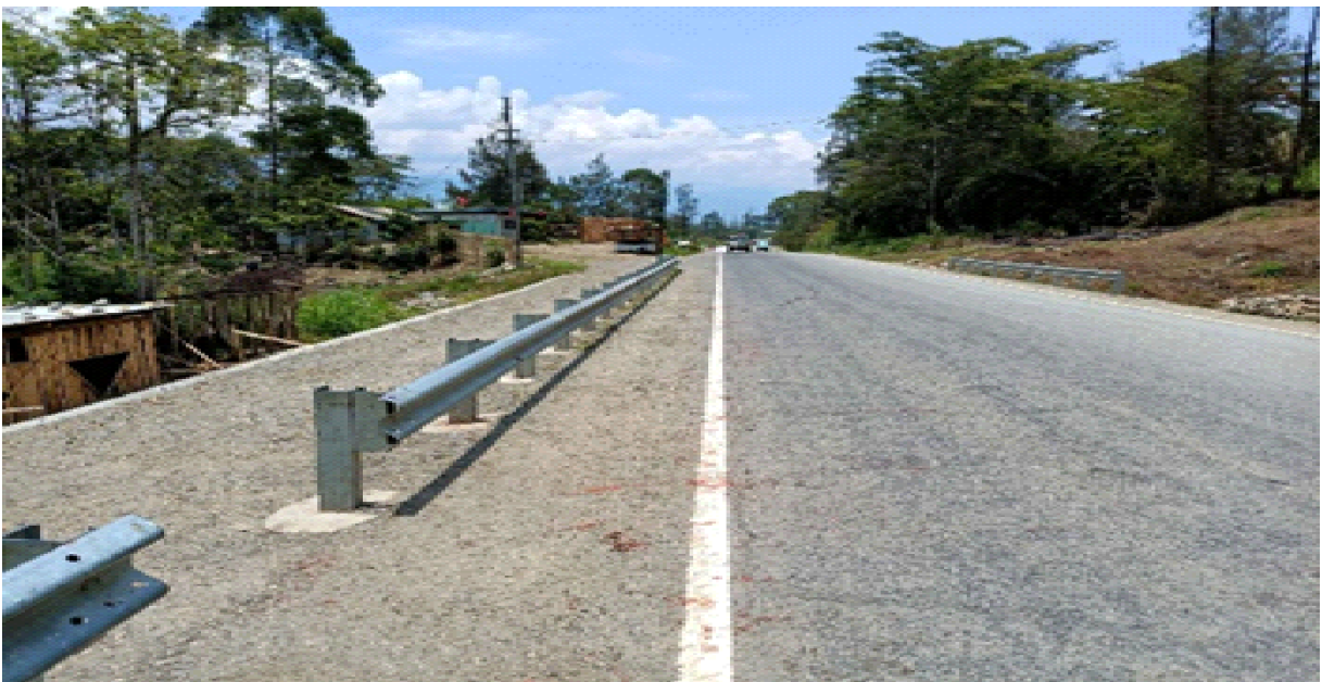
Photo 12: Guard Installation and Line Marking, Migende Section, Highlands Highway to improve safety standards
