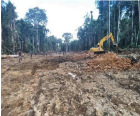
Excavation for Drainage Works
