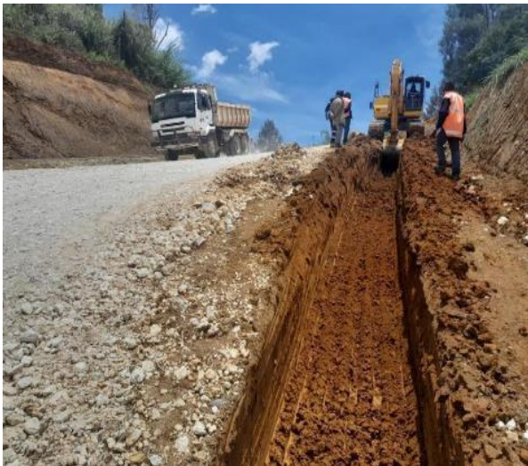
Photo 66: Rehabilitation, Upgrading and Sealing of Halimbu-Idauwi, Hela Province.
