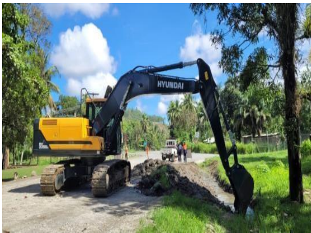
Photo 90: Upgrading and Sealing-Bulolo Junction-Hidden Valley Junction, Bulolo District.
