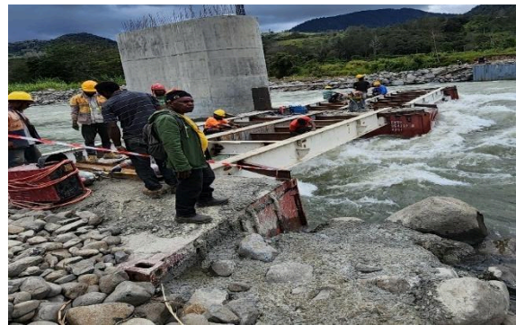
Photo 63: Site Works on the Construction of Yalo Bridge 150m span, Compact 200 Double Single Reinforced Bailey Bridge, Ialibu District.
