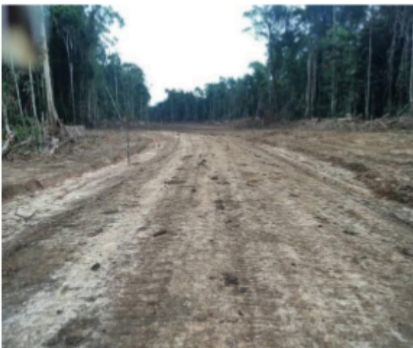
Clearing of New Cut Road
