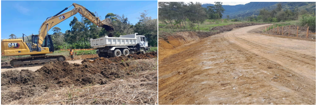
Photo 87: Pavement Rehabilitation and Associated Drainage Works, Wapenamanda District
