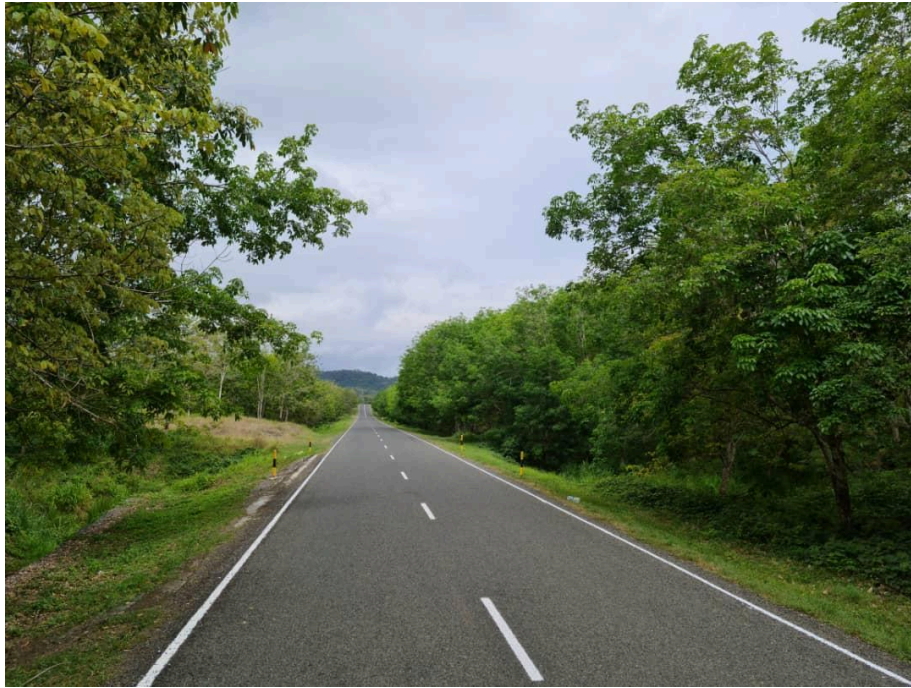
Photo 26: Hiritano Highway, Central Province, Southern Region
