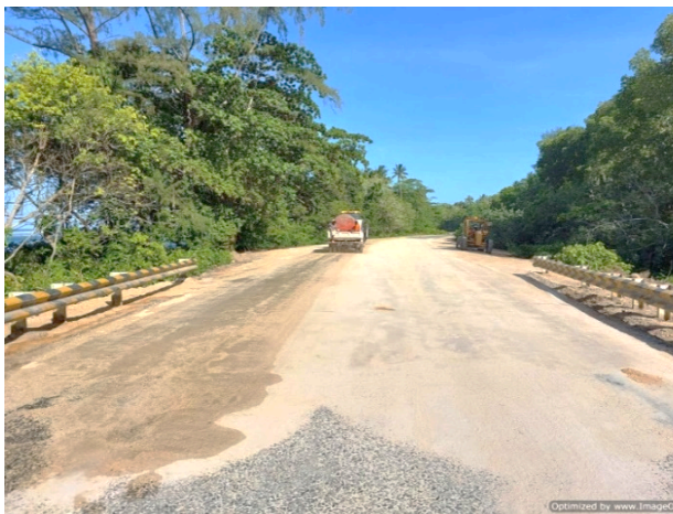
Photo 34: Various works on the Boluminsky Highway under TSSP.
