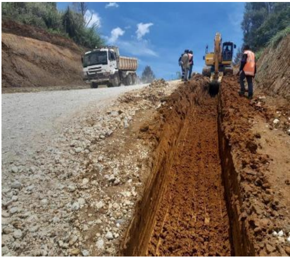
Photo 40: Rehabilitation, Upgrading and Sealing of Halimbu-Idauwi, Hela Province.
