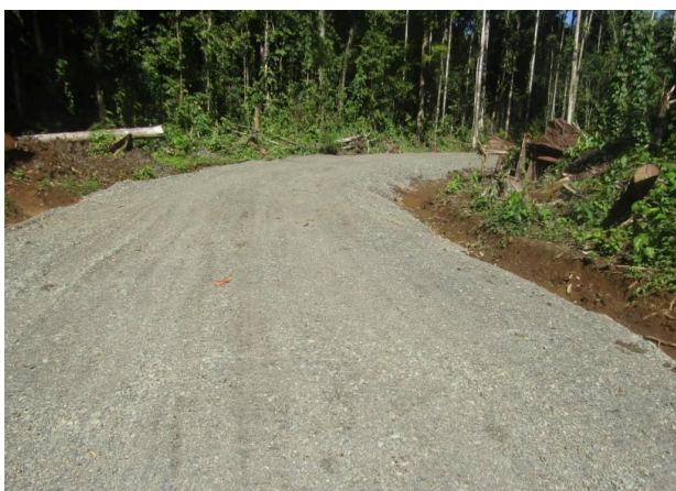
Photo 51: Recently constructed Sections of the Central-Milne Bay Missing Link Road.
