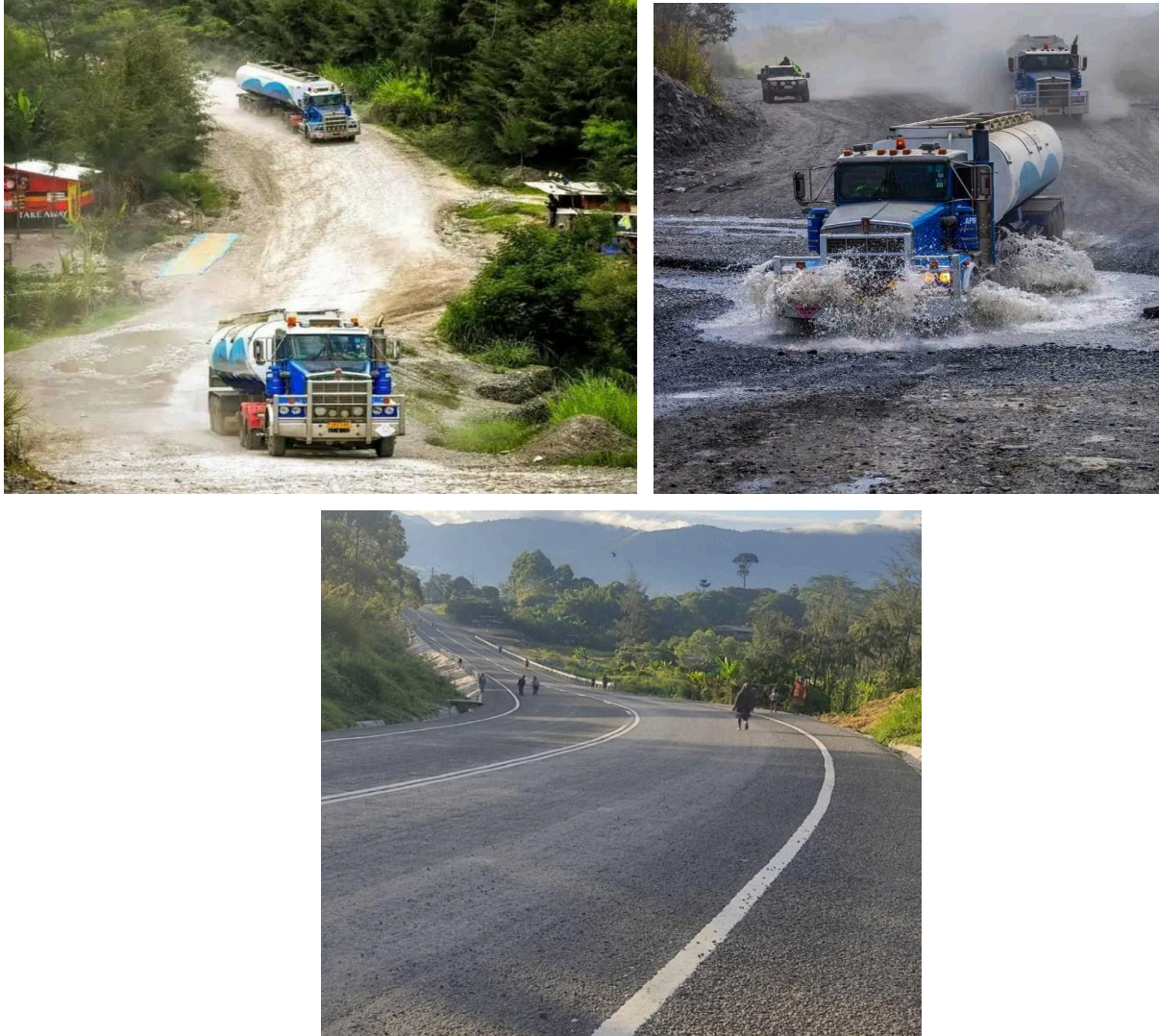
Photo 62: Left Photo show condition of the Wara Tamba Section (Simbu), Highlands Highway. The Photo below show it is after it has been upgraded and improved under SHHIP Tranche 1.
