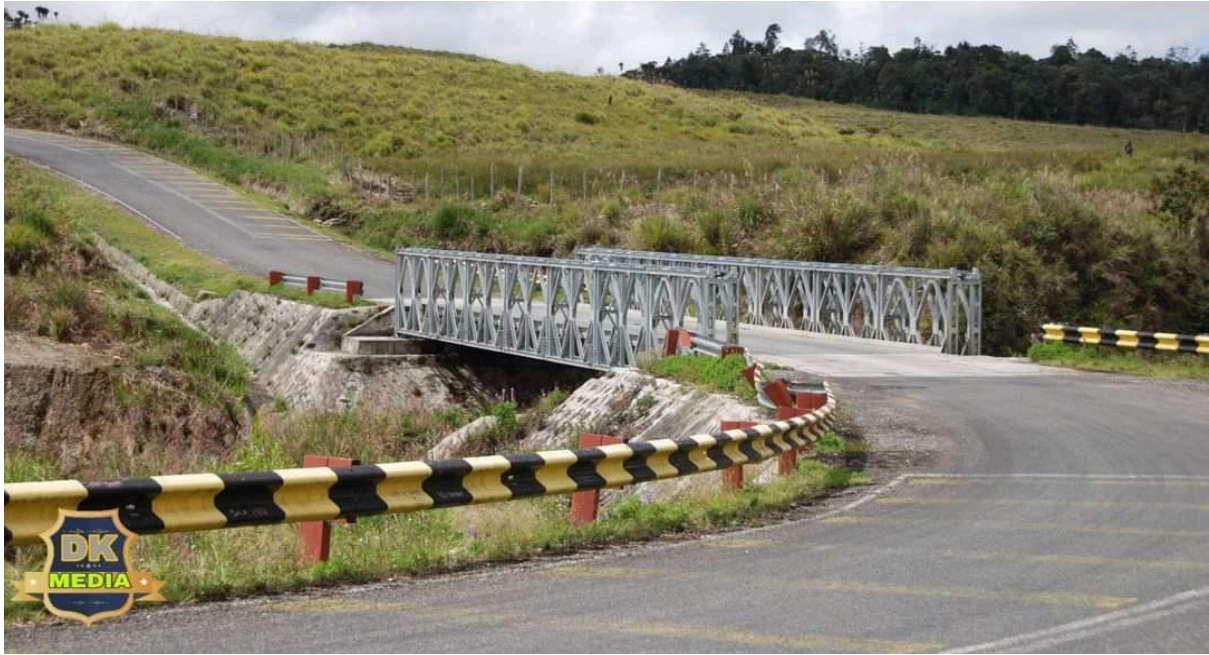
Photo 85: Rural Bailey Bridge Standard delivered on Tambul-Nebilyer District Rural Road under the Multi-Year Rural Bridging Program with United Pacific Bridges Ltd.
