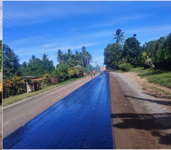
Photo 109: Pavement Repair and Reseal with Associate Drainage Works On 17.18 Km Section of the 30km Seal Section between DoWH Junction and Bola Junction along Talasea Road.
