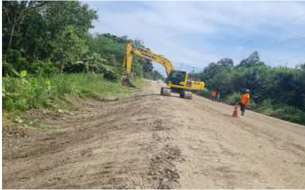
Photo 28: Pavement Construction, Yakura Bridge - Ono Mountain Section, Ramu Highway
