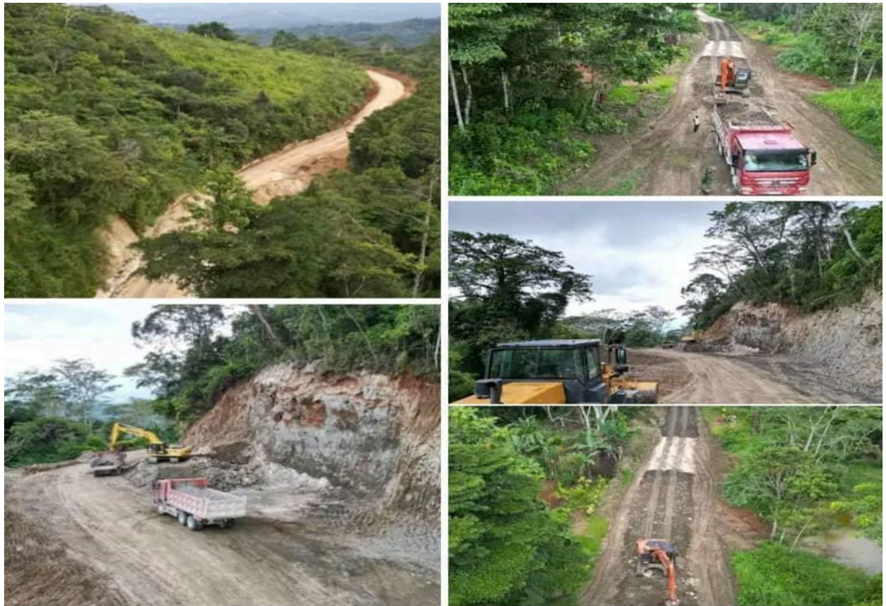
Photo 52: Current work on the construction of the Lae-Finschaffien Missing Link Highway.
