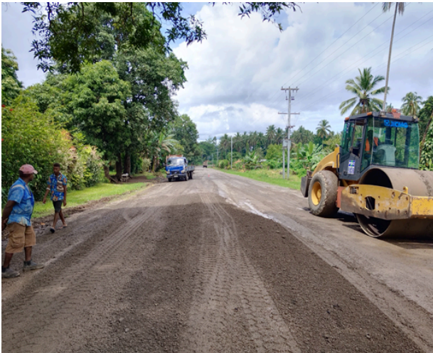
Photo 64: Pavement Repair and Reseal with Associate Drainage Works On 17.18 Km Section of the 30km Seal Section between DoWH Junction and Bola Junction along Talasea Road.
