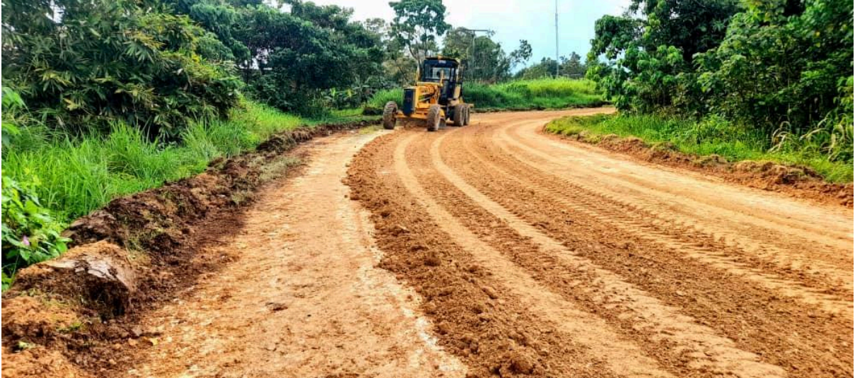
Photo 43: Upgrading road leading to Palmalmal Town-Pomi District
