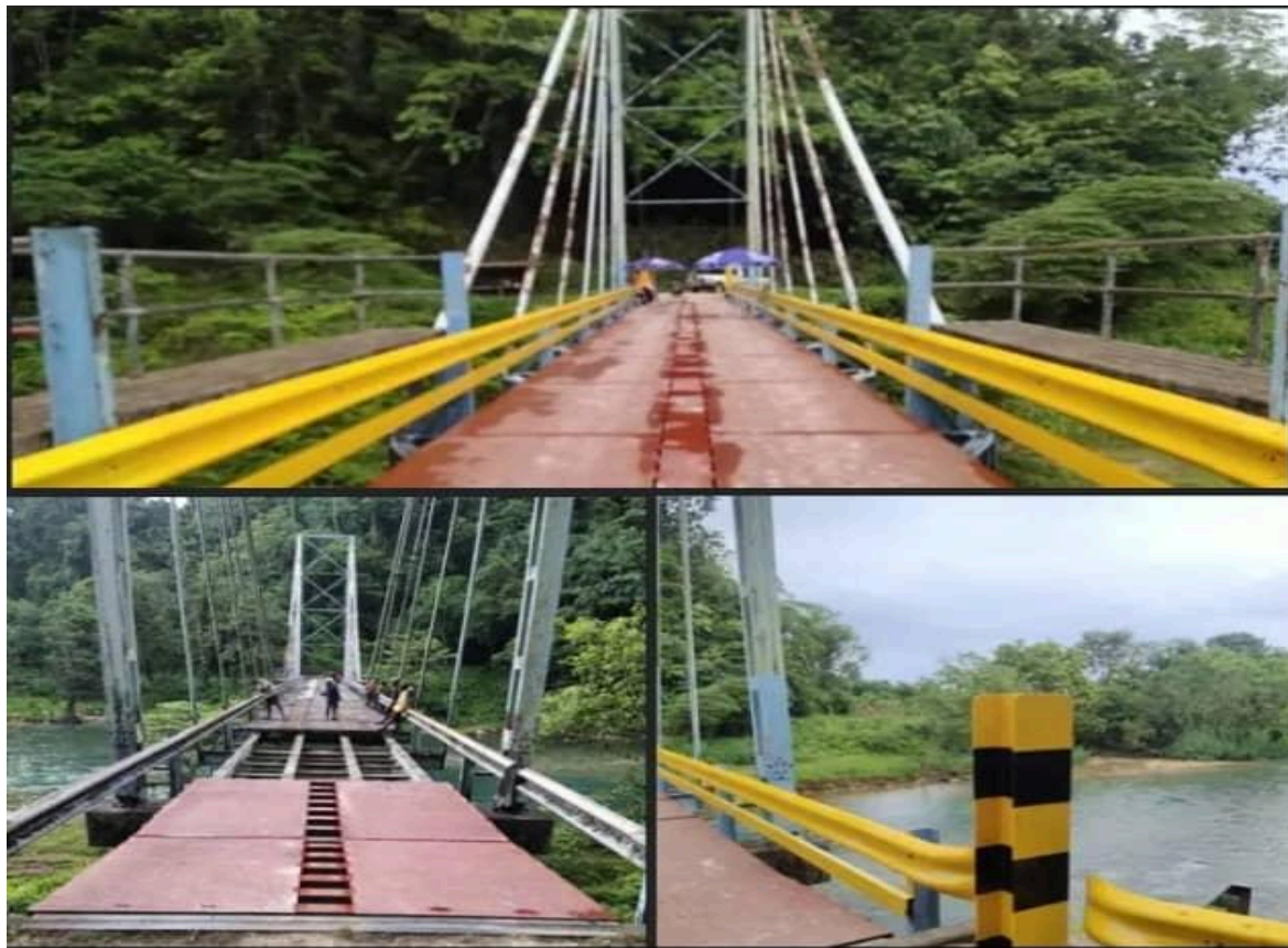
Photo 86: Matale Bridge, Central Pomio LLG, East New Britain Province.
