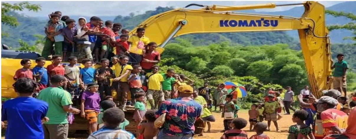
Photo 37: One of the Machines supplied under Japanese Aid on Trans-National Highway
