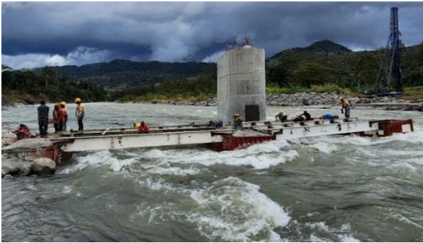
Photo 63: Site Works on the Construction of Yalo Bridge 150m span, Compact 200 Double Single Reinforced Bailey Bridge, Ialibu District.
