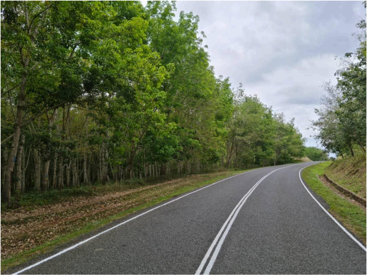
Photo 107: Hiritano Highway, Central Province, Southern Region
