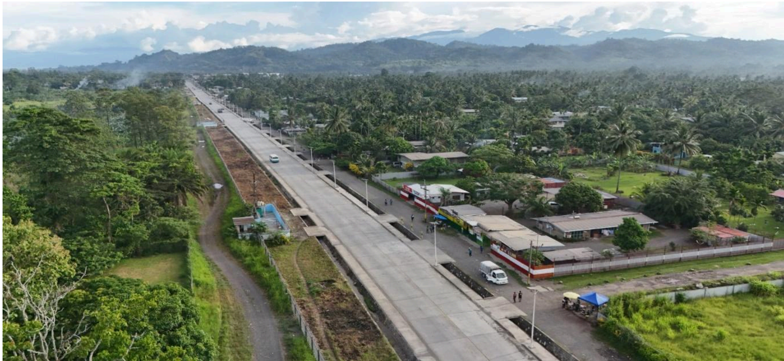
Photo 81: Lae city upgraded to Concrete and Climate Resilience surfaces.
