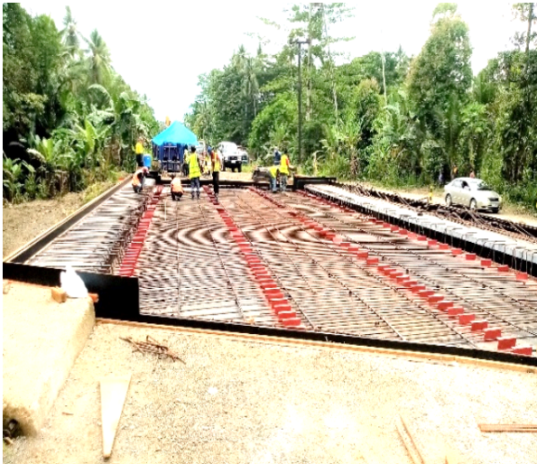
Photo 35: Reconstruction of Dewala Bridge, Magi Highway, under TSSP
