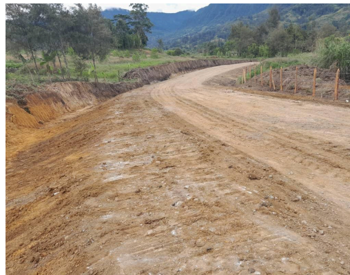
Photo 96: Pavement Rehabilitation and Associated Drainage Works, Wapenamanda District
