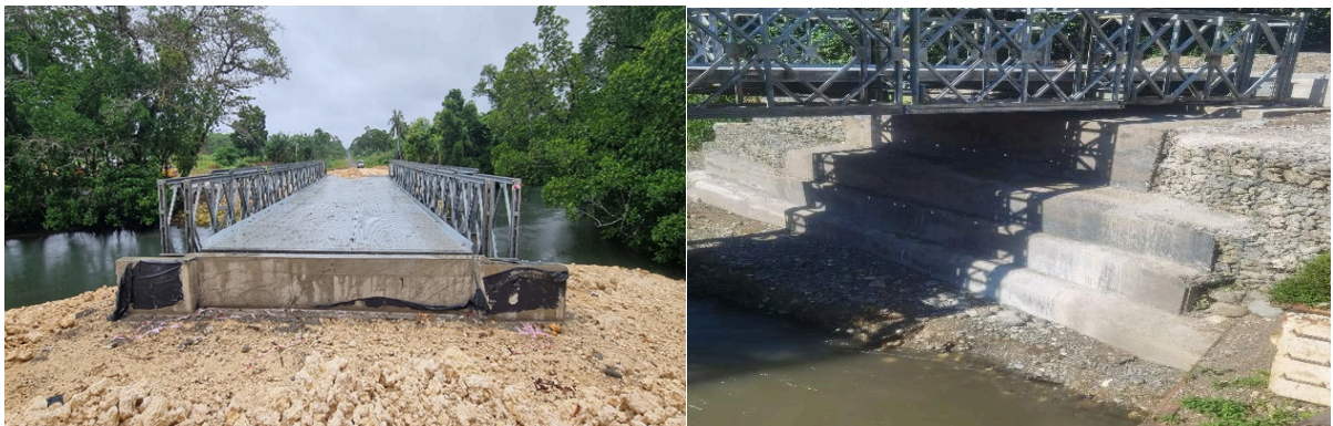
Photo 49: Replacing Girity Log Bridge with Compact 200 Bailey -New Britain Highway
