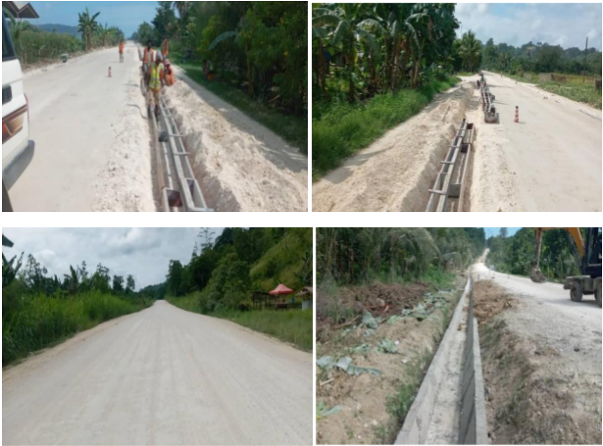
Photo 98: Construction in Progress Sawmill-DPI Station, Sepik Coastal Highway-Phase 2
