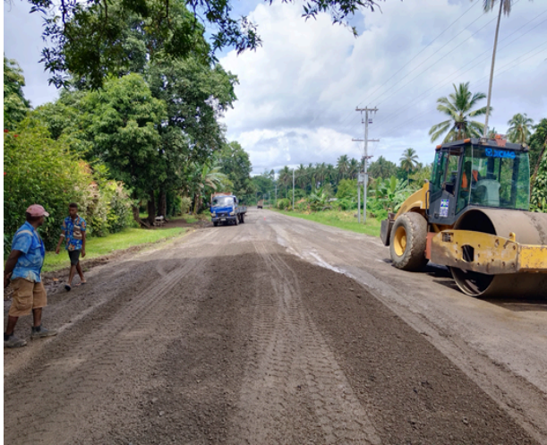
Photo 109: Pavement Repair and Reseal with Associate Drainage Works On 17.18 Km Section of the 30km Seal Section between DoWH Junction and Bola Junction along Talasea Road.
