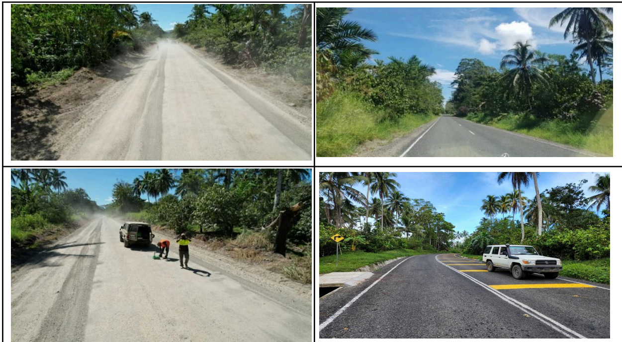
Photo 27: Before and After photos Reconstruction, Upgrading and Sealing from Buin Kangu Wharf to Toimonapu (60km) of the Aropa Coastal Road in the Autonomous Region of Bougainville
