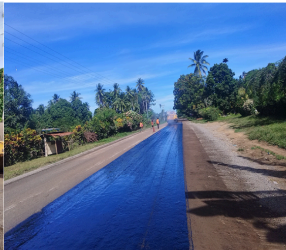
Photo 64: Pavement Repair and Reseal with Associate Drainage Works On 17.18 Km Section of the 30km Seal Section between DoWH Junction and Bola Junction along Talasea Road.
